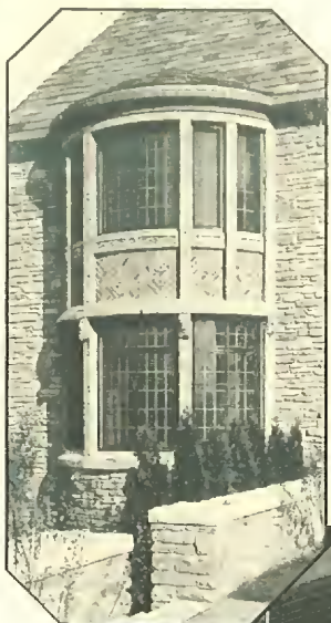
These stationary screens (right) on outside of inswinging casements, are bowed to the contour of the bay.
